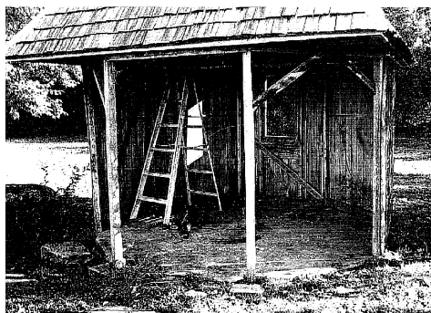
Figure 17. Interior of the summer house, showing constructional details.
