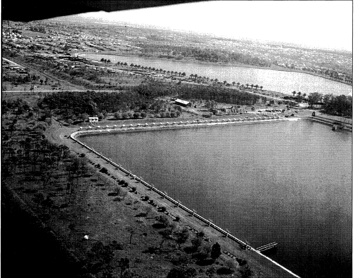
Figure 7: The solar grating arrays in 1953, looking south-west. The E-W arm consisted of thirty-two 6-ft paraboloids while the N-S arm had sixteen 10-ft paraboloids. Aperture synthesis was achieved by combining the Fourier components from each arm (courtesy ATNF Historic Photographic Archive: B3475-1).
