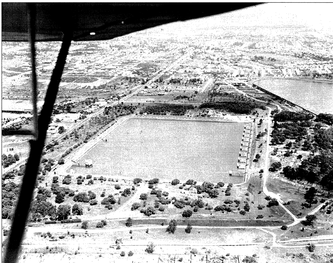
Figure 3: Aerial photograph, looking south, of the eastern reservoir at Potts Hill. Eventually, radio telescopes and associated huts were located along the southern and eastern margins of the reservoir, and across the extended area of flat land in the foreground, to the north of the reservoir (courtesy ATNF Historic Photographic Archive: B3253-1).
