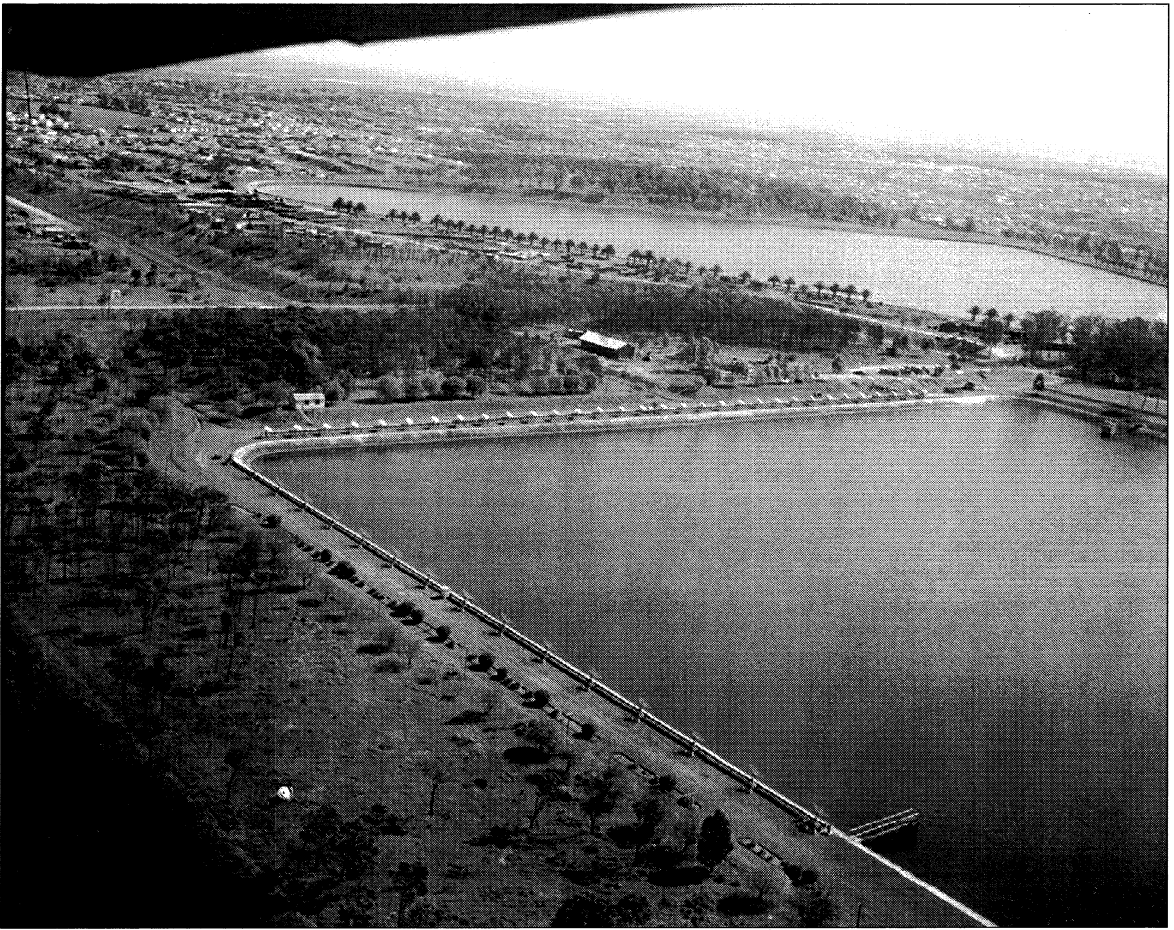
Figure 6: View looking southwest across the two Potts Hill water reservoirs in 1953, showing Christiansen's solar grating arrays along the banks of the eastern reservoir. The E-W array consisted of thirty-two elements and the nearer N-S array just sixteen elements (ATNF Historic Photographic Archive: 3475-1).
