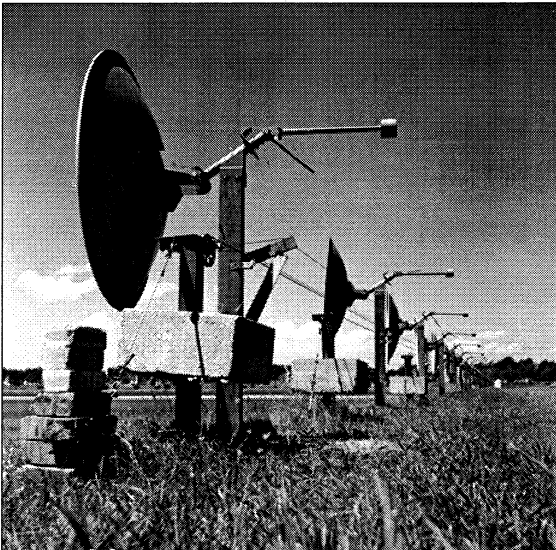
Figure 7: Close-up, looking east, showing the E-W grating array (ATNF Historic Photographic Archive: B2976-1).
