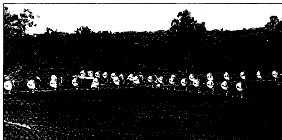
Figure 11: The completed Stanford 9.2 cm cross-antenna interferometer (after Bracewell, 2005: 75).
