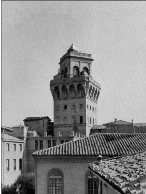
Figure 1: This photograph from the early 1950s shows the Observatory tower, which rises over the rooftops of the main campus of the University of Bologna. The dome visible in the foreground on the terrace of the second-to-last floor of the tower (which has since been replaced by a lift) housed the Steinheil telescope. The dome to the left of the terrace, on the same floor, is the one that was built in 1850 to hold the Ertel & Sohn meridian circle and was restored in the late 1900s (courtesy: Archive of the Department of Astronomy, University of Bologna).
