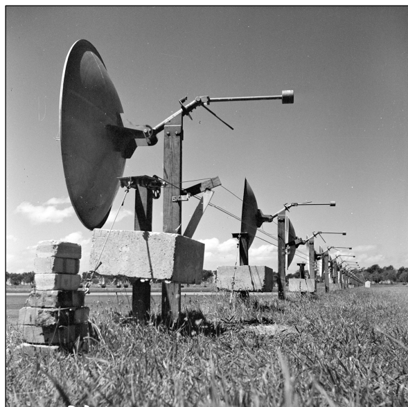
Figure 3: Another view of the east-west array, showing the bracing weights for the open-wire transmission lines. The parabolas were equatorially mounted, with the declination set for the given day. The right ascension was changed in 15 minute steps using holes and a locking pin on the mount (courtesy ATNF Historic Photographic Archive).
