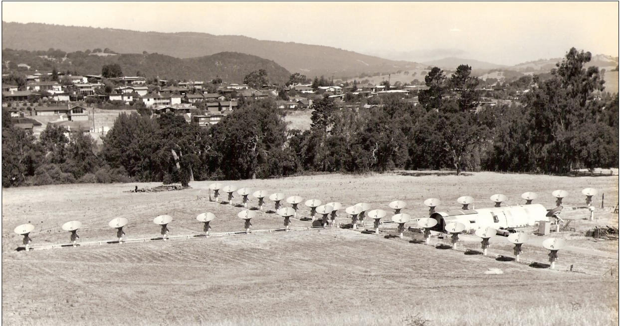
Figure 6: Panoramic view of the 9.1 cm Stanford Microwave Spectro-heliograph Antenna (courtesy: Stanford University Photographic Department, Negative No. 9448).
