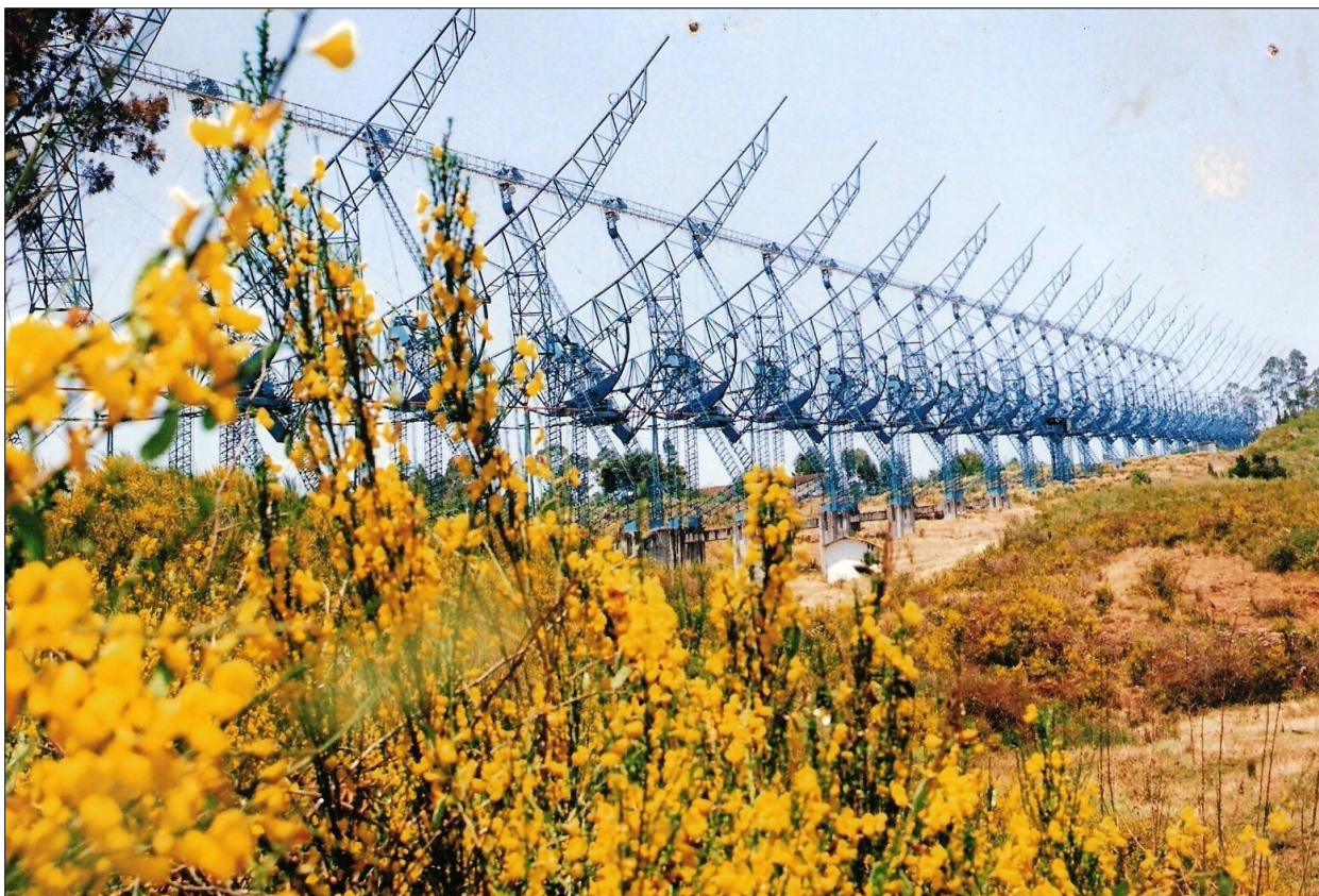
Figure 9: The Ooty Radio Telescope, a 530m \times 30m cylindrical parabolic antenna in Southern India.
