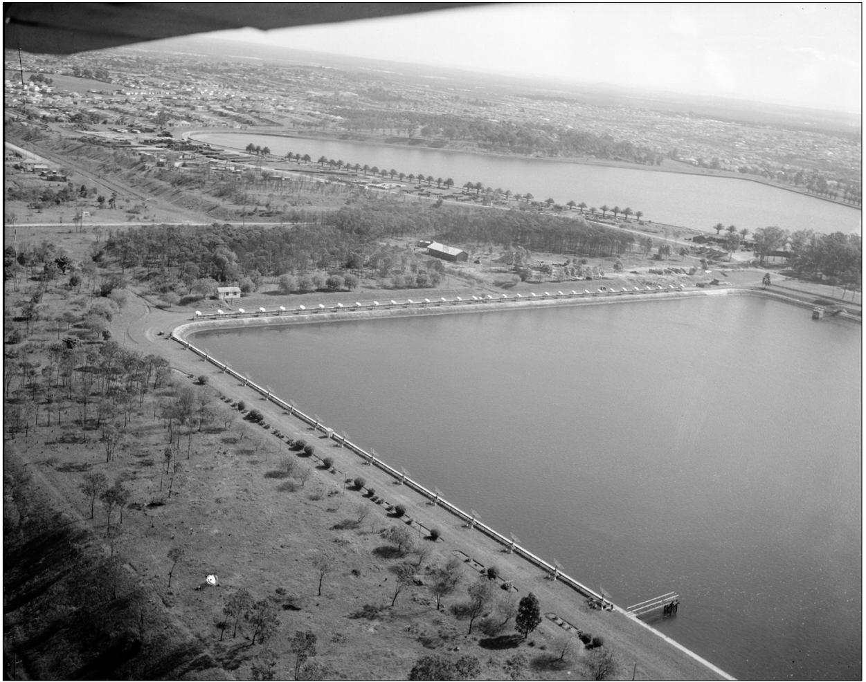
Figure 2: Aerial view looking southwest across the two water supply reservoirs at Potts Hill. The 32 antennas comprising the east-west solar grating array can be seen on the southern edge of the foreground reservoir, and the 16-element north-south grating array is clearly visible along the eastern edge of this same reservoir (courtesy: ATNF Historic Photographic Archive, 3475-1).
