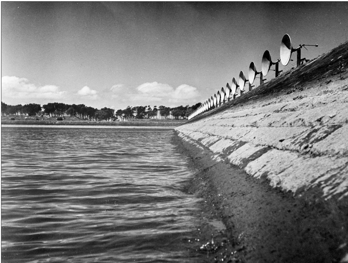
Figure 1: View looking east showing the east-west grating interferometer on the southern bank of one of the two Sydney water supply reservoirs at Potts Hill (courtesy: ATNF Historic Photographic Archive, B2638-2).
