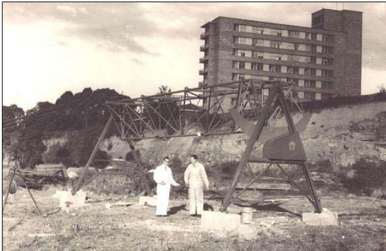
Figure 3: The beginning of the Cross. Terry Butcher and Alec Little with the prototype EW module at the old St. Leonards brick pit in Sydney. The prominent building in the background is part of the Royal North Shore Hospital.
