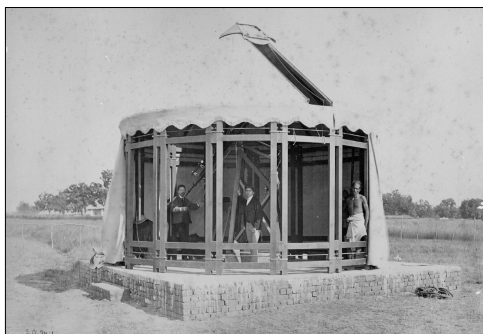
Figure 6: The dome that housed the Steinheil refractor at the Italian station in Muddapur, India. Pietro Tacchini is on the left, by the Tauber spectroscope from Palermo, which was adapted to the telescope (private archive).
