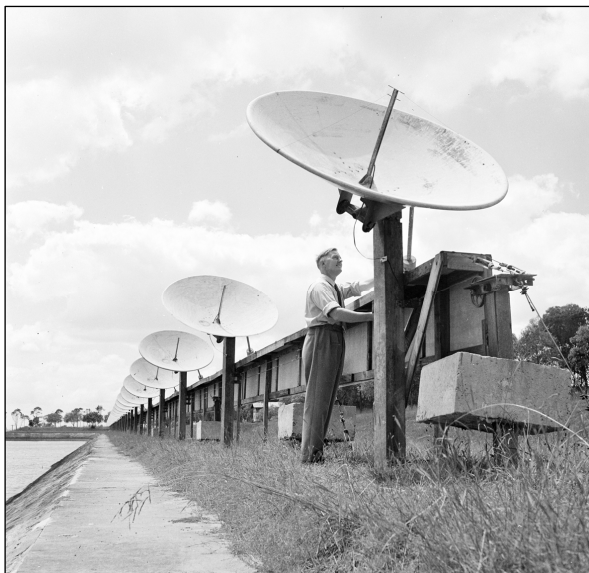
Figure 2: View looking east showing W.N. Christiansen and the 32-element solar grating array at Potts Hill in the western suburbs of Sydney (courtesy ATNF Historic Photographic Archive).
