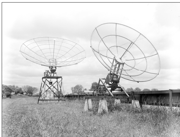
Figure 22: The prototype of the larger 5.8m aerial (left) that would be used in the new crossed array at Fleurs being tested at Potts Hill in 1956 adjacent to the north-south grating array (courtesy ATNF Historical Photographic Archive).
