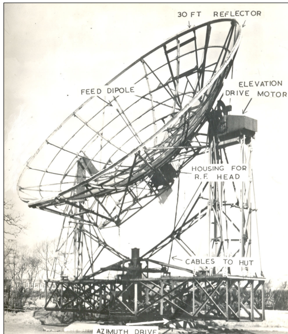
Figure 3: The 30-ft telescope at Jodrell Bank used for the first H I observations in 1954. This antenna was originally sited on the south coast of England during WWII where it was used for anti-aircraft surveillance (after Davies, Ph.D. thesis, University of Manchester, 1956).
