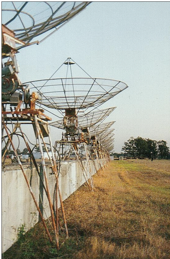
Figure 49: A view looking south along the N-S arm of the decommissioned Chris Cross showing rusting antennas (courtesy John Leahy).
