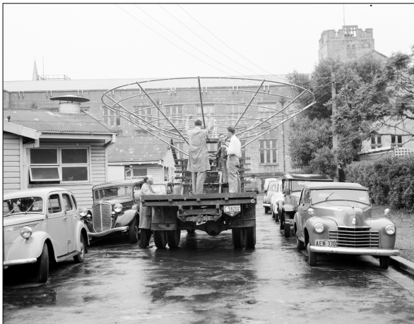
Figure 8: Loading the Chris Cross test antenna onto a truck at the RP Workshop, ready for its transfer to Potts Hill field station (courtesy ATNF Historic Photographic Archive: B3858-3).
