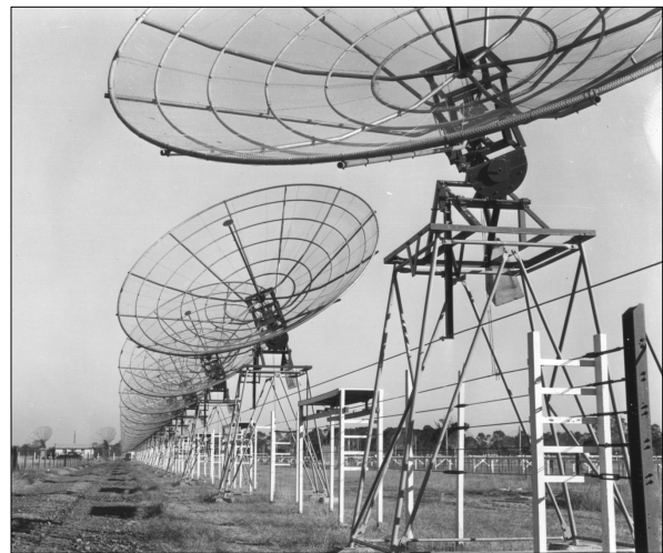
Figure 19: View of the newly-completed Chris Cross, looking south along the N-S arm. Note the five vertically-stacked twin feeder lines, and the steel cable used to drive the array (courtesy ATNF Historic Photographic Archive: B5192-5).
