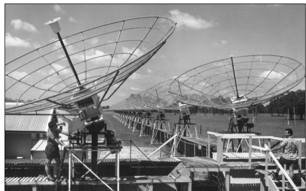
Figure 20: View looking south along the N-S arm, near the centre of the Cross. Note the superstructure erected to protect the feeder lines from the elements (courtesy ATNF Historic Photographic Archive: B9097-12).
