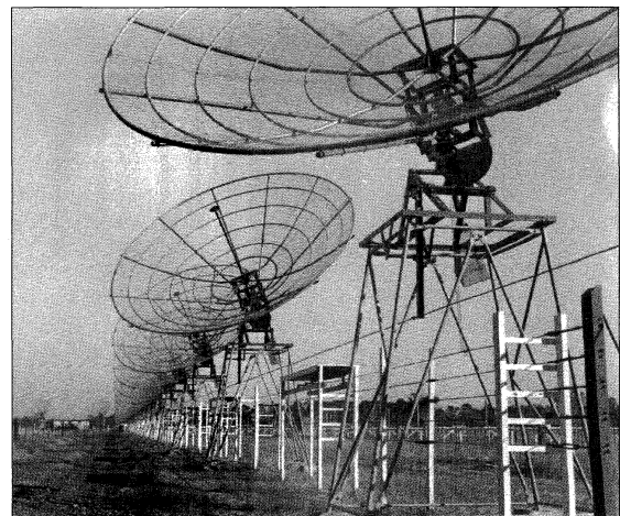
Figure 19: View of the newly-completed Chris Cross, looking south along the N-S arm. Note the five vertically-stacked twin feeder lines, and the steel cable used to drive the array (courtesy ATNF Historic Photographic Archive: B5192-5).
