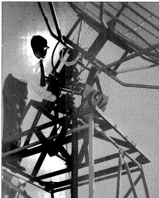
Figure 12: Close-up of the equatorial mounting, showing the hour angle circle, the white declination sector and the ratchet wheel used to drive the aerial when observing the Sun (courtesy ATNF Historic Photographic Archive: B5804-4).
