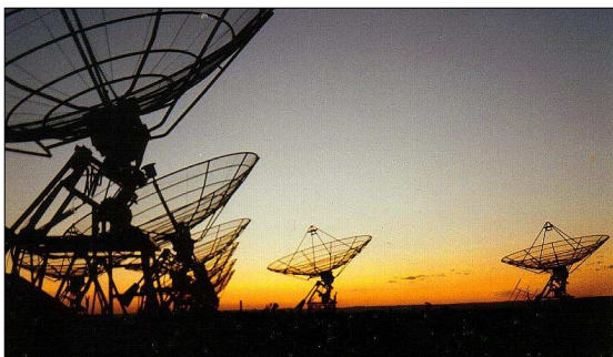
Figure 2: View of the central part of the Chris Cross, looking west at sunset. This array comprised E-W and N-S arms each with 32 steerable parabolic antennas of 5.8m diameter. This was the world's first crossed-grating interferometer and it was used to produce daily isophote maps of solar emission at 1423 MHz (photography courtesy John Leahy).
