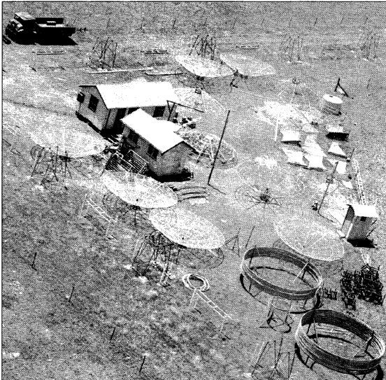
Figure 13: Aerial view showing huts, cylindrical frames and the antenna assembly area of the new Chris Cross, located very close to the central point of the Cross (courtesy ATNF Historic Photographic Archive: B5042-2).
