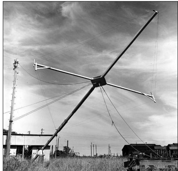
Figure 13: Photograph of the rhombic aerial and pulley system with Bill Rowe standing nearby. In the background to the right are the railway locomotive shunting sheds (courtesy: ATNF Historical Photographic Archive).
