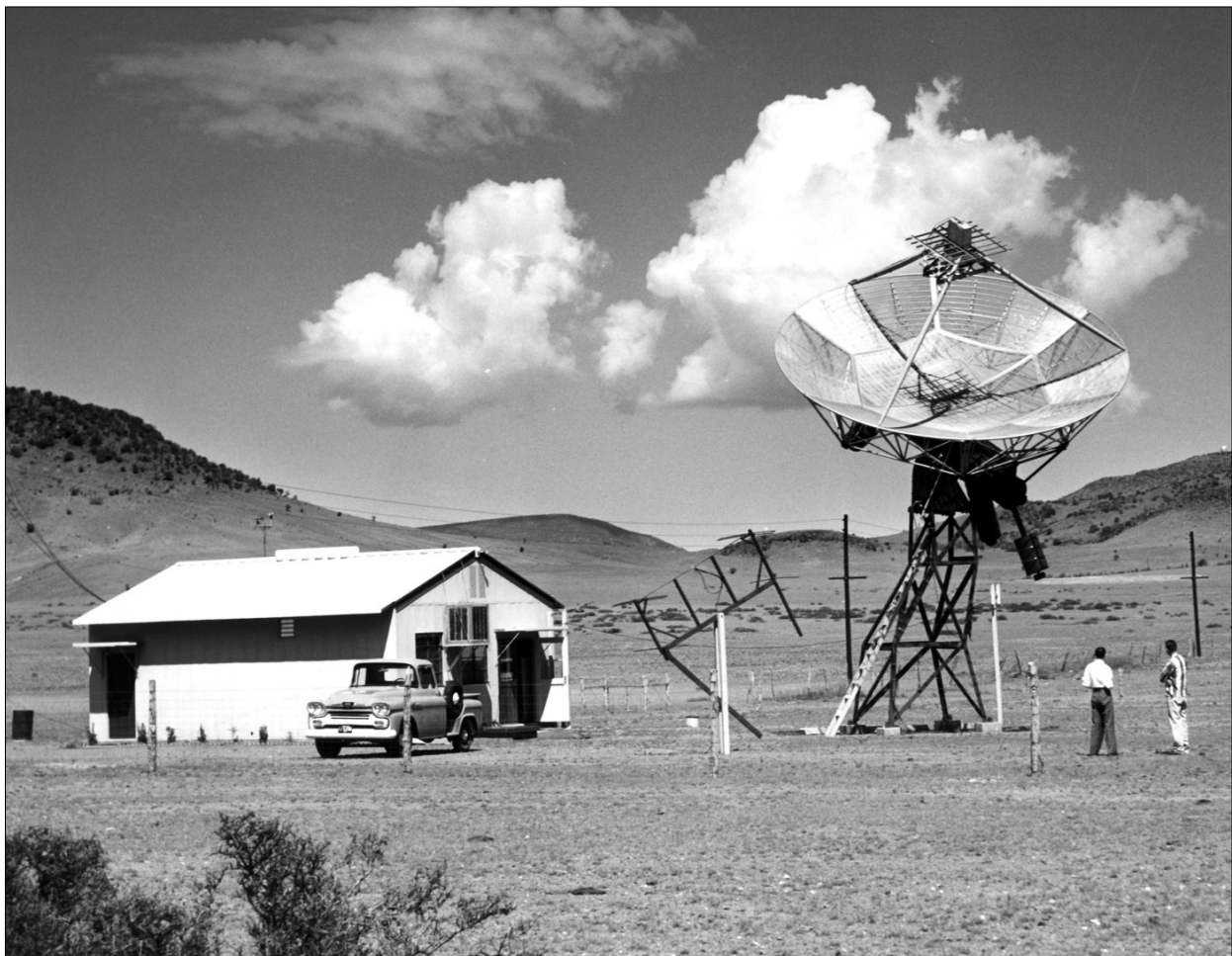
Figure 1: The 28-ft. diameter antenna and solar laboratory building as they appeared in 1958. The small antenna near the center of the picture, consisting of two dipoles with reflectors, was used with a 70 MHz fixed-frequency receiver and chart recorder. It provided a real-time indication of the state of solar activity, which was useful since the outputs of the spectral receivers could not be examined until the film was developed. Note that the dome of the McDonald Observatory, approximately 4 miles distant, is just visible on the horizon near the right-hand edge of the picture (Photograph supplied by A. Maxwell, Harvard College Observatory).
