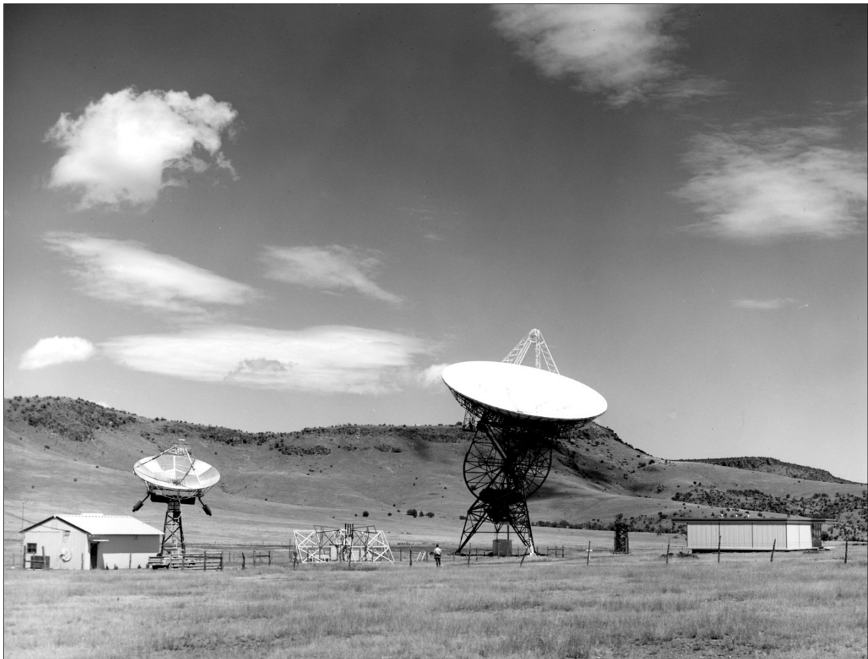
Figure 9: The site in 1964. From left to right: the solar laboratory, the 28-ft. antenna, the 25-50 and 50-100 MHz dipoles and the 70 MHz monitoring antenna, the 85-ft. antenna, an extendable tower for access to the focus of the 85-ft. antenna, and the new laboratory building for the 85-ft. antenna. The figure near the 85-ft. antenna is laboratory assistant C. Murray (Photograph supplied by A. Maxwell, Harvard College Observatory).
