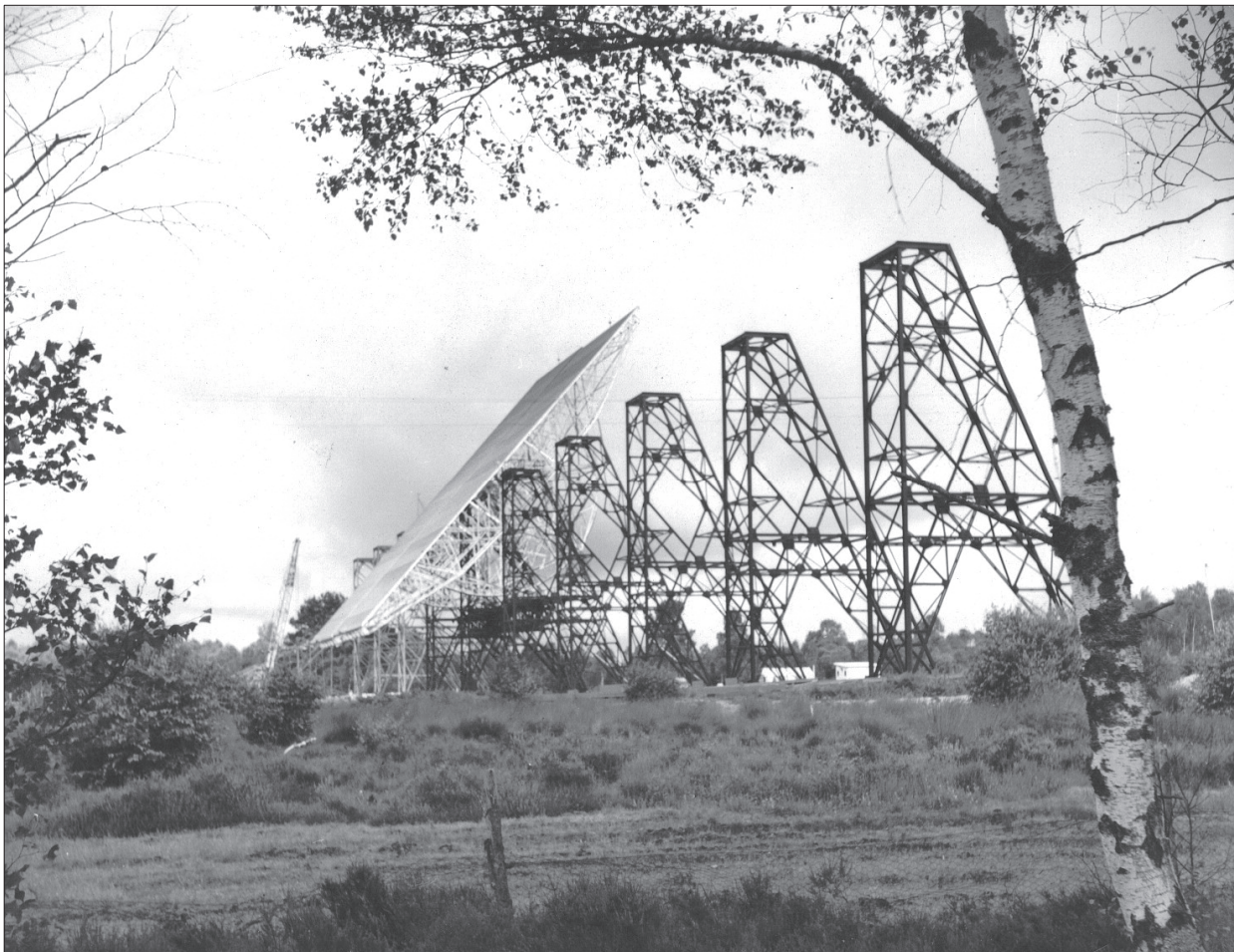
Figure 9: The fully-tiltable mirror during construction.
