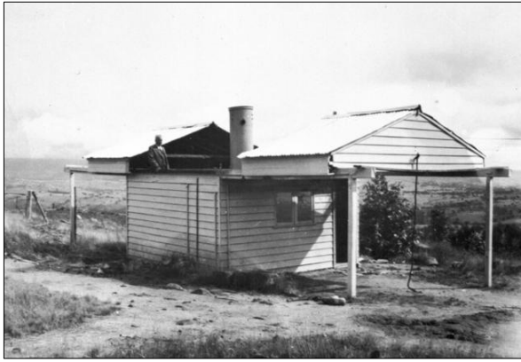
Figure 6: The Catts Telescope roll-off roof observatory at MSO (courtesy: Mount Stromlo and Siding Spring Observatories).
