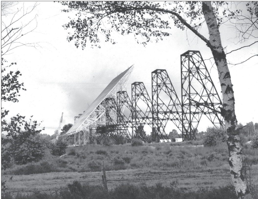
Figure 9: The fully-tiltable mirror during construction.
