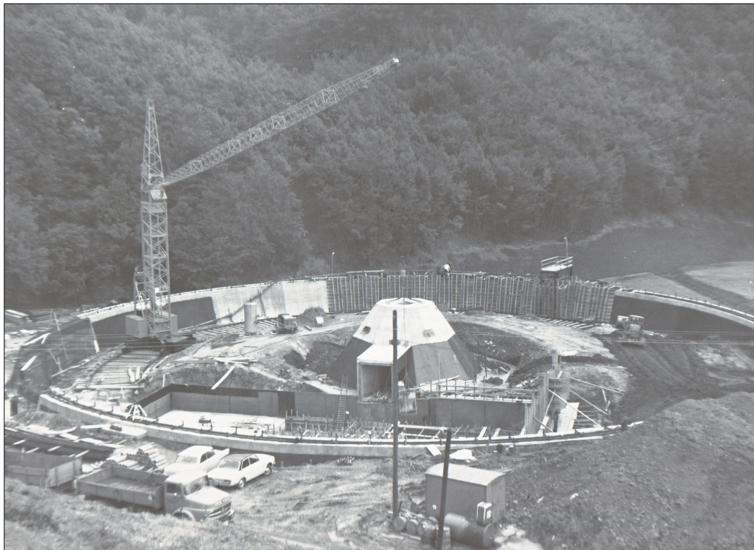
Figure 2: The foundations for the 100-m radio telescope in the construction phase (1968).
