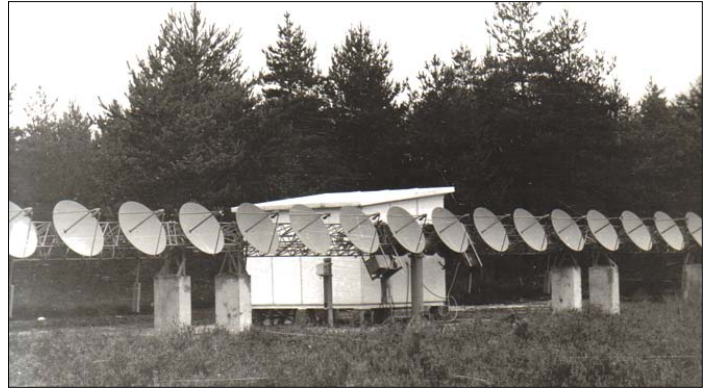
Figure 7: The Nançay 9300 MHz E-W array.
