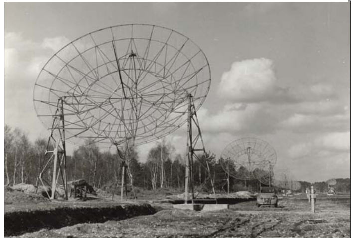
Figure 8: The 8 parabolic antennas of the N-S array.
