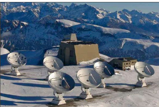
Figure 11: A recent view of the IRAM interferometer on Plateau de Bure, with its 6×15-m antennas. The large shelter in the background is used for antenna construction and maintenance (courtesy: IRAM).
