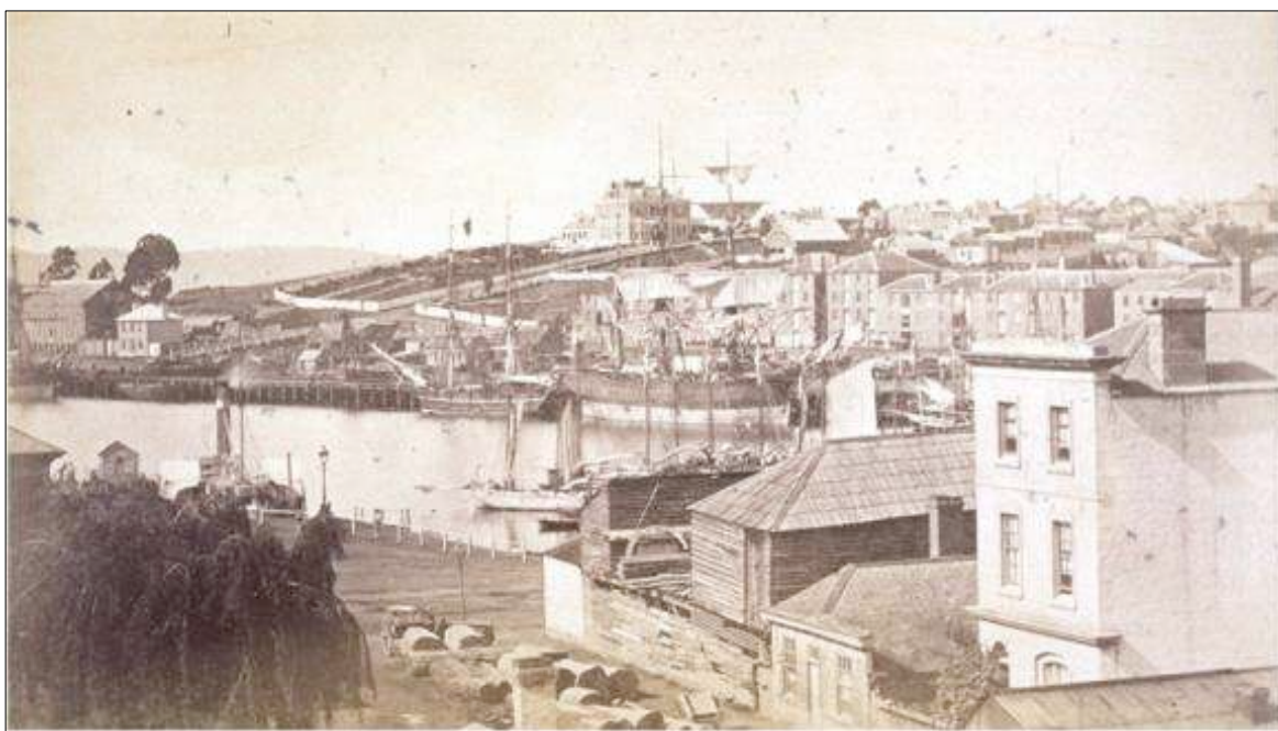
Figure 6: An 1878 photograph titled "New wharf ...", showing Lenna and the time ball mast (courtesy: W. L. Crowther Library, Tasmanian Archive and Heritage Office).
