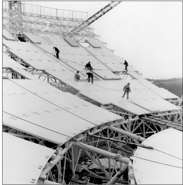
Figure 6: Assembly of the panels on the partly-constructed reflector.
