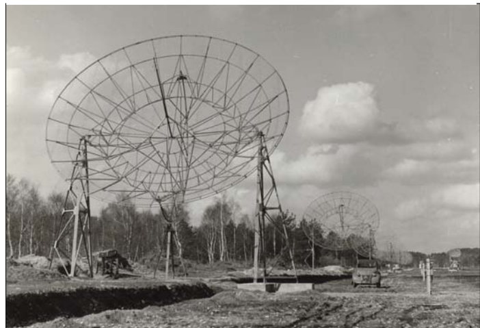
Figure 8: The 8 parabolic antennas of the N-S array.
