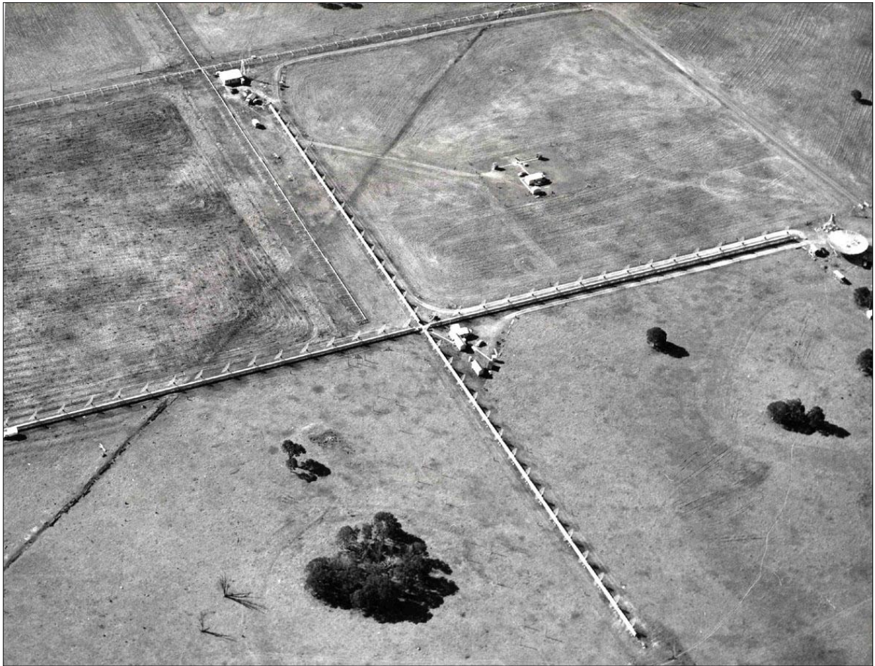
Figure 2: An aerial view of the Chris Cross at Fleurs looking north-east, with the 18-m Antenna (far right) under construction at the eastern end of the E-W arm of the Cross (courtesy: ATNF Historic Photographic Archive).
