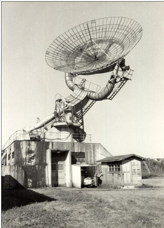
Figure 10: The 10-m equatorially-mounted dish erected at the TAO in 1953, which was used to monitor solar radio emission at 200 and 3000 MHz (courtesy: National Astronomical Observatory of Japan Archives).
