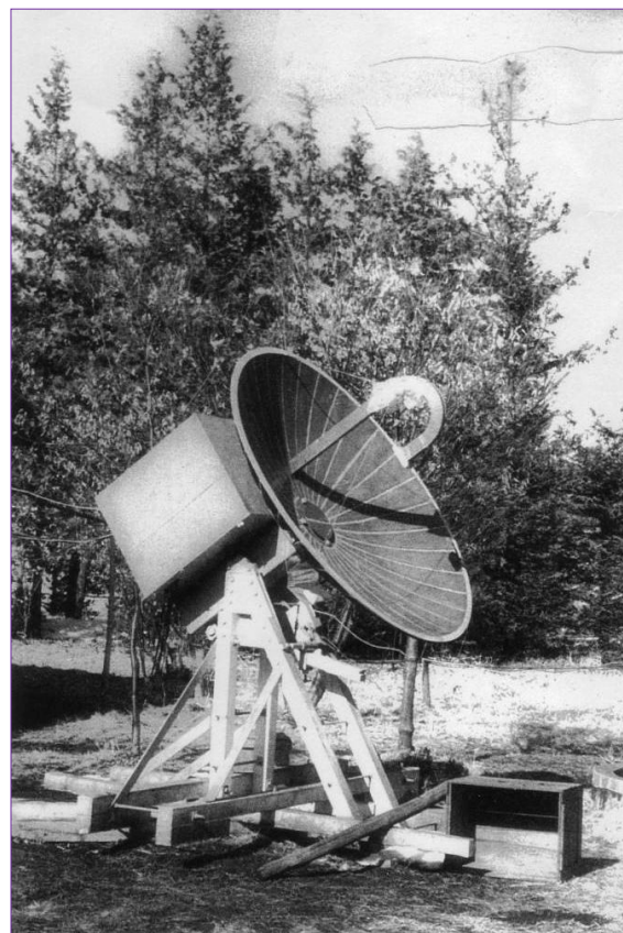
Figure 8: The radio telescope at Mitaka, completed by Kenji Akabane, which used Shimoda’s original parabolic reflector.
