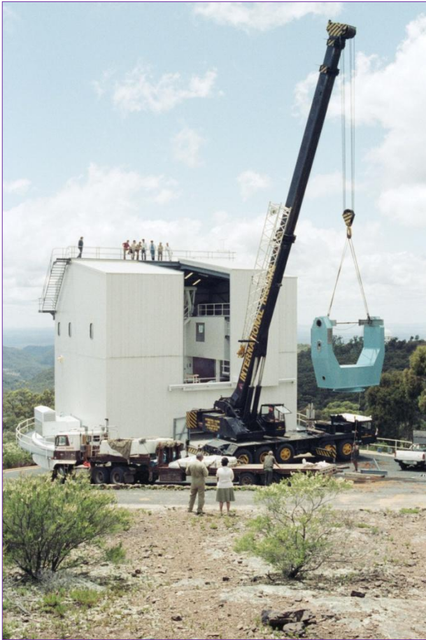
Figure 23 (top left ): The telescope fork being lifted into the newly-completed building.
