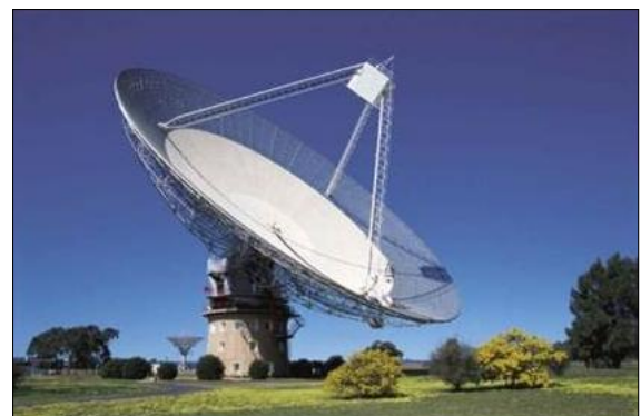
Figure 8: The 64-m Parkes Radio Telescope (photograph: K.I. Kellermann).
