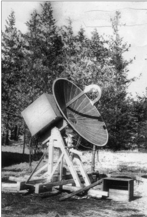
Figure 8: The new 3 GHz radio telescope that used Shimoda's old parabolic dish (courtesy: K. Akabane).
