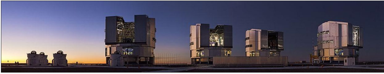
Figure 10: ESO's Very Large Telescope at Cerro Paranal, showing the buildings that house the four 8.2-m telescopes, which can be used individually or as an interferometer ( en.wikipedia.org ).
