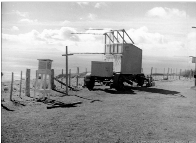
Figure 15: The mobile radio telescope on the Greenwood farm at Pakiri Hill in June 1948. The cabin mounted on the trailer could swivel in azimuth to observe sources rising at different declinations along the horizon (courtesy: Stanley family).
