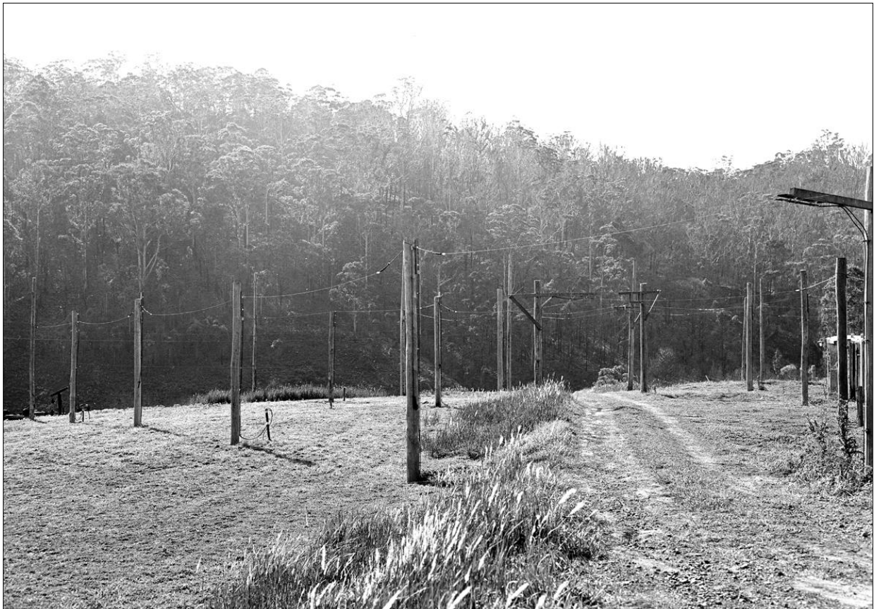
Figure 5: The low frequency radio telescopes at Hornsby Valley consisted of posts that were used to support the dipoles, with the ground serving as a reflector (courtesy CASS RAIA: B2802-5).
