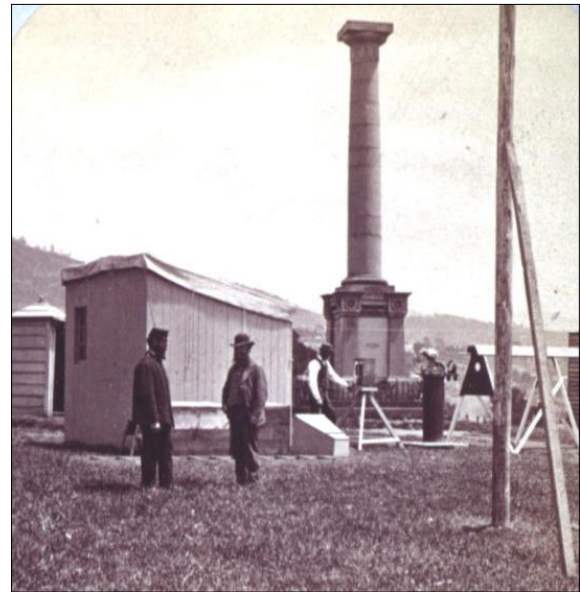
Figure 6: One of a stereo pair of photographs of part of the Hobart 1874 transit station, showing (left to right) the 'Transit House', heliostat drive, heliostat pier, and part of the wooden superstructure protecting the measuring rod (leading to the 'Photographic House'). In the background is the 'soldiers' monument' (courtesy: W.L. Crowther Library, Tasmania Archives and Heritage Office, ADRI:AUTAS001125299032).
