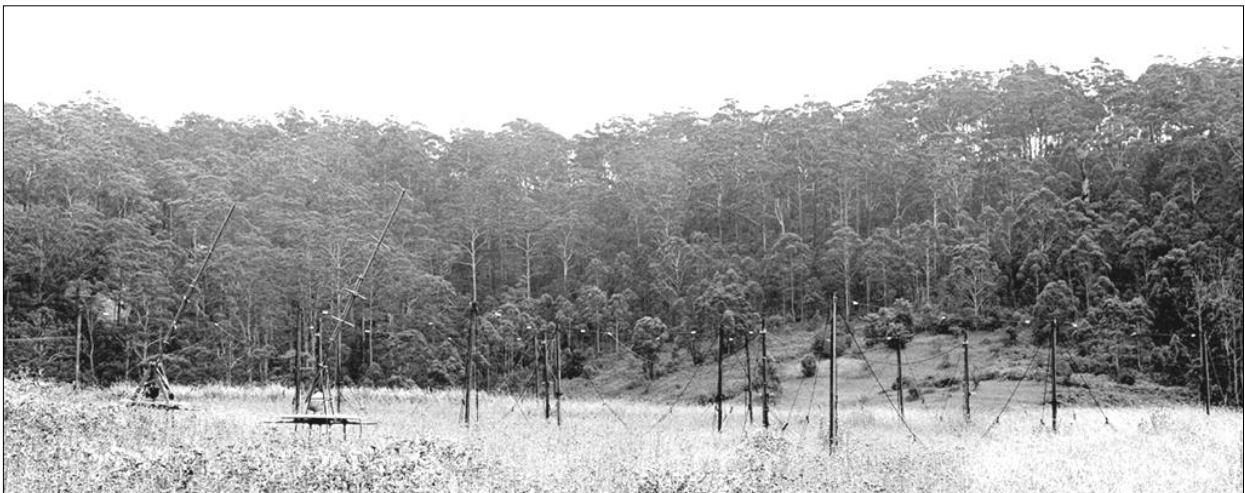
Figure 40: The 60 MHz and 85 MHz Yagi antennas (on the left) and the 19.8 MHz rhombic antenna (centre and right) used by Ruby Payne-Scott for her solar observations in 1948 (courtesy: CSIRO RAIA B1266-2).
