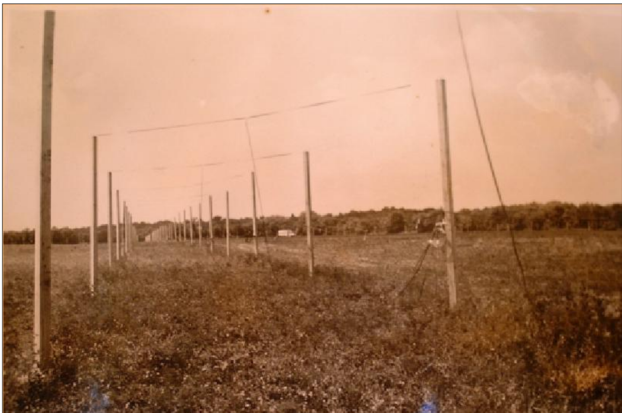
Figure 31: A view looking along one of the arms of the 22 MHz Mills Cross at Seneca, Maryland. Each arm was 624 metres long, and contained 66 dipoles (courtesy: Carnegie Institution of Washington).
