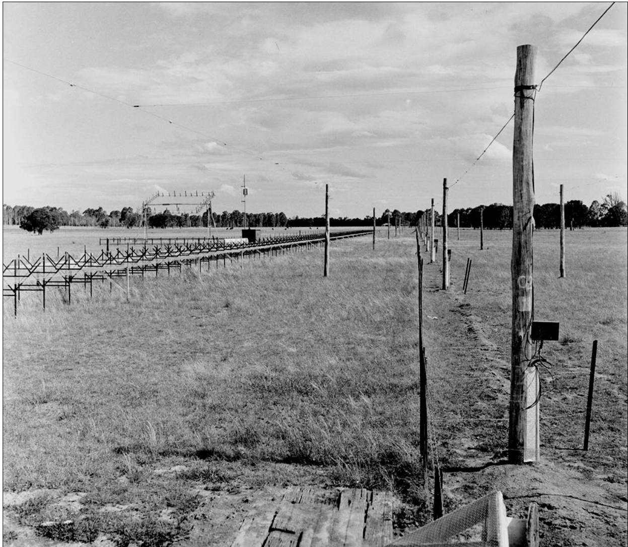
Figure 9: A view looking south along the N-S arm of the Shain Cross. To the left is part of the south arm of the Mills Cross and a broadside array that was used to investigate the angular sizes of discrete sources (courtesy: CASS RAIA: B3868-19).
