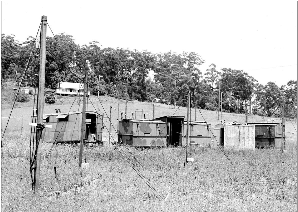
Figure 3: A close-up of the assemblage of huts, trailers, poles and wiring associated with the Moon bounce experiment (courtesy: CSIRO RAIA B1266-5).
