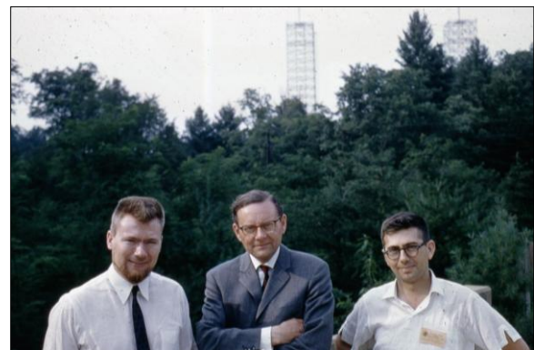
Figure 10: Professor Biermann (centre) with two technicians visiting the Sugar Grove radio telescope project in West Virginia in 1961. Note the construction towers in the background (courtesy: Hastings Pawsey and Miller Goss).
