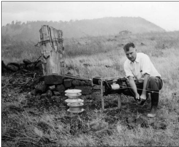
Figure 10: Reber with a winch. This is almost certainly at the eastern end of Antenna 4 (courtesy: ANRAO).
