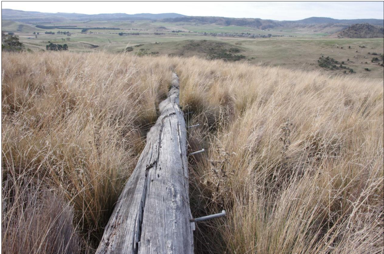
Figure 13: The western pole for Antenna 3, in 2015. It stood until about 2002, when it finally fell (photograph: Martin George).
