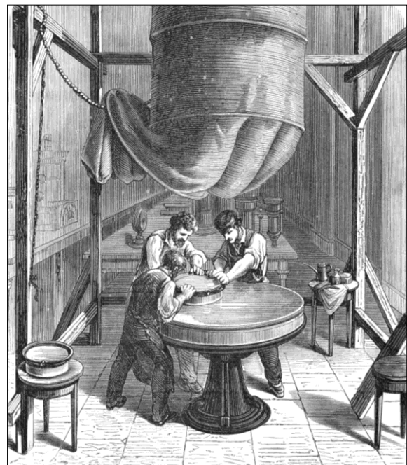
Figure 32: For diameters up to about 40 cm Foucault worked the mirror against a glass 'ball'. The increased forces needed to figure larger sizes were counteracted by employing several workmen or by suspending the upper piece from springs. Final polishing was accomplished with smaller tools, as illustrated here for the 120-cm mirror worked by Foucault's pupil Adolphe Martin in the 1870s. A decade earlier Foucault (1864a) had thought it "... extremely likely ..." that machine polishing would be needed for a mirror this big, and indeed the 120-cm mirror was not a success. The mirror is shown being worked in the Meridian Room of the Paris Observatory. The vertical cloth tube indicates that it was tested making use of the zenithal well that pierces the height of the Observatory (after: L'illustration , No 1668, 117 (1875); author's collection).
