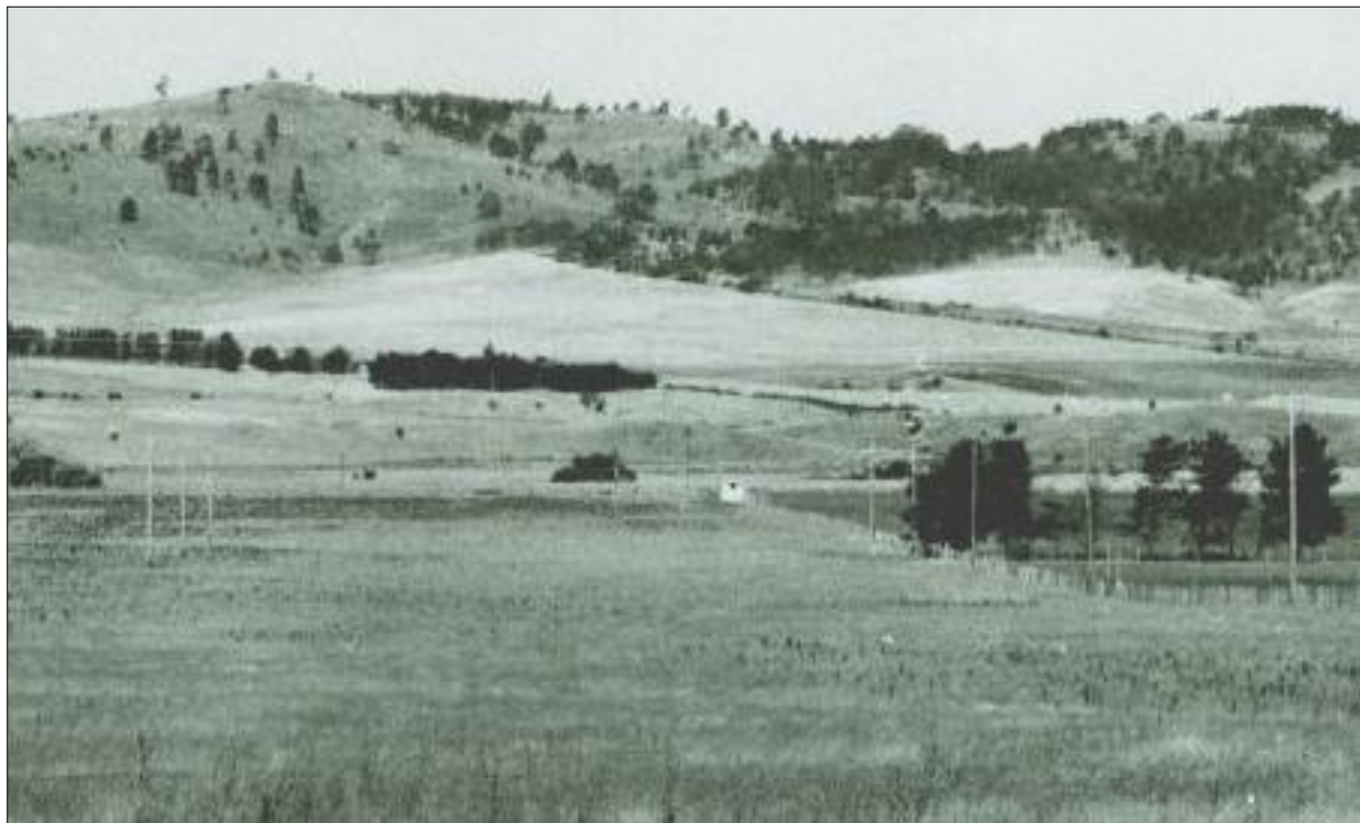
Figure 3: A panoramic view looking east south east showing parts of the Richmond arrays (the three poles on the left and the five poles along the fence-line on the right), and the hut (just right of centre) containing the receiving equipment (after Bessell, 1963).
