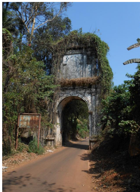
Figure 19: The Arch of Conception in Old Goa (photograph: R.C. Kapoor, 24 February 2016).
