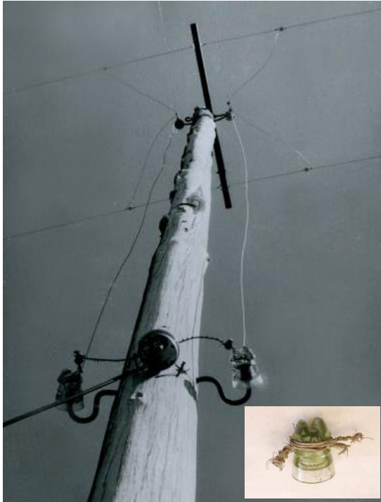
Figure 8: One of the telegraph poles at Richmond, with a close up of an insulator shown in the inset photograph (after Bessell, 1963).
