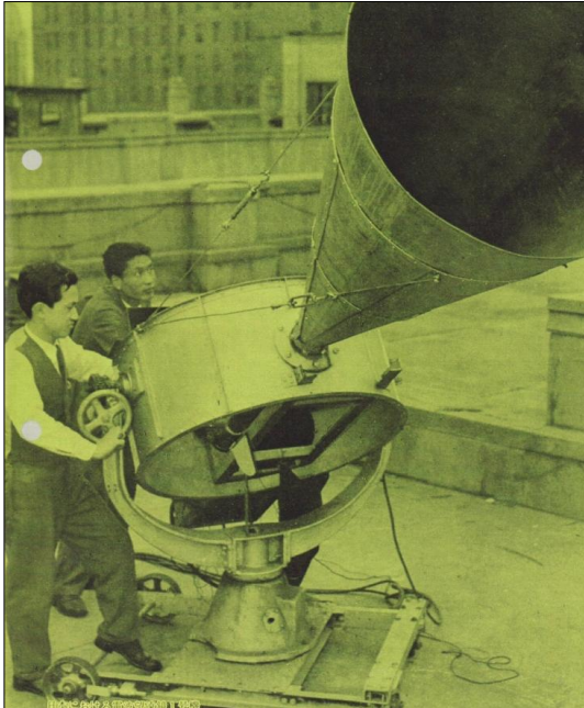
Figure 4: Oda (left) and Takakura (right) with their simple horn radio telescope at Osaka University in November 1949 (after Takakura 1985: front cover).
