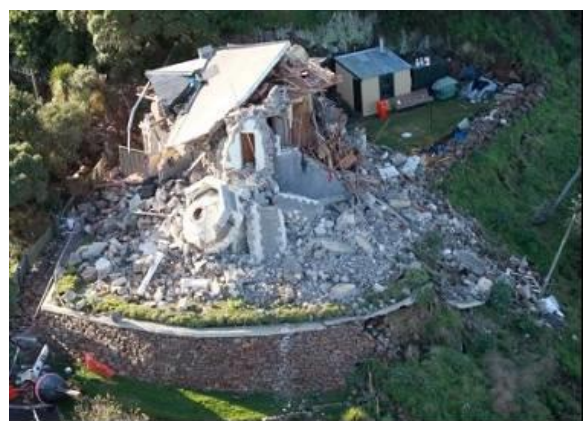
Figure 9: A photograph taken on 18 June 2011, five days after the collapse of the Lyttelton Time Ball Tower ( www.stuff.co.nz/national/christchurch-earthquake/5145289/June-13-earthquakes-Morale-costs-get-a-shake-up ).
