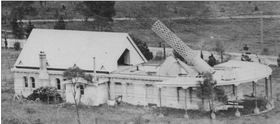
Figure 17: At Melbourne Observatory there was the roll-off roof observatory built for the 48-in (1.22-m) Great Melbourne Telescope (courtesy: Harley Wood).
