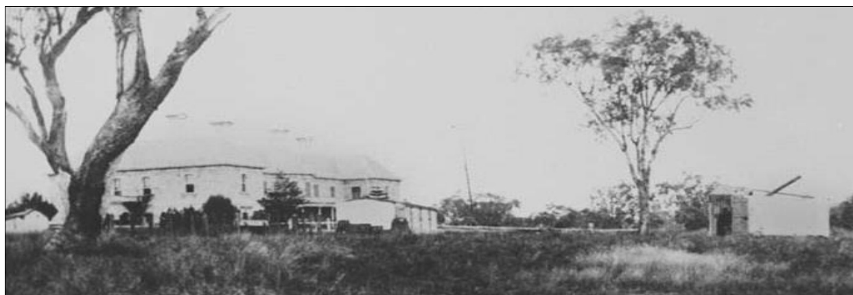
Figure 5: Jimbour House (left) and some of the temporary observatories of the British transit party. On the far right (with one of the telescopes protruding) are the observatories containing Peek's and Morris' refractors, while the transit telescope was housed in the building in the middle of the photograph. The location of the observatory that housed Darwin's refractor is not specified (after van Roode, 2011).
