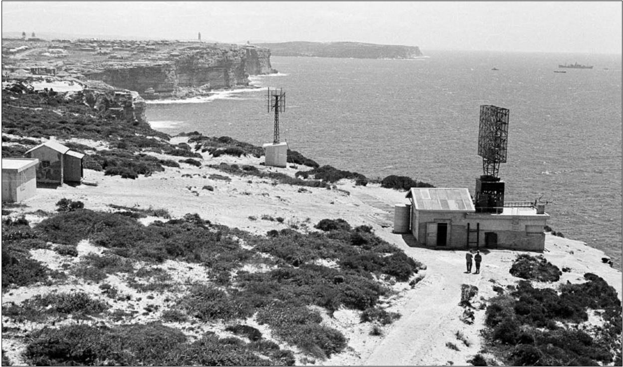
Figure 2: A view looking north showing the Dover Heights radar station in the foreground, and beyond it North Head (where there also was a radar station) and the entrance to Sydney Harbour. The radar antenna on the roof of the cliff-side blockhouse was used initially for solar radio astronomy, then it was removed and the Yagi antennas used by Bolton, Stanley and Slee were installed on the roof of the blockhouse (courtesy: CSIRO Radio Astronomy Image Archive (henceforth CRAIA) B81-1).
