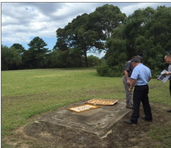
Figure 47: A recent view at Potts Hill of the concrete pad that supported the ex-Georges Height experimental radar antenna (photograph: Harry Wendt).
