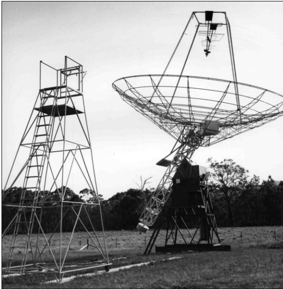
Figure 46: The new 10-m dish with the old ex-Potts radar antenna mounting that was installed at Dapto Field Station in 1963 (courtesy: CRAIA, 004032).
