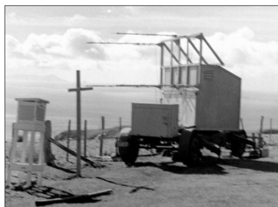
Figure 11: The mobile radio telescope on the Greenwood farm at Pakiri Hill in June 1948. The cabin mounted on the trailer could swivel in azimuth to observe sources rising at different declinations along the horizon (courtesy: Stanley family).
