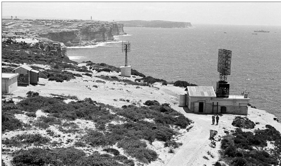
Figure 2: A view looking north showing the Dover Heights radar station in the foreground, and beyond it North Head (where there also was a radar station) and the entrance to Sydney Harbour. The radar antenna on the roof of the cliff-side blockhouse was used initially for solar radio astronomy, then it was removed and the Yagi antennas used by Bolton, Stanley and Slee were installed on the roof of the blockhouse (courtesy: CSIRO Radio Astronomy Image Archive (henceforth CRAIA) B81-1).
