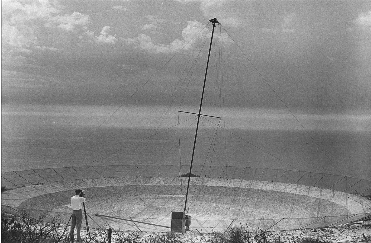
Figure 24: The enlarged concrete-coated 80-ft HitGA in September 1953, with Gordon Stanley using a theodolite to record the position of the aerial mast (courtesy: RAIA B3150-2).
