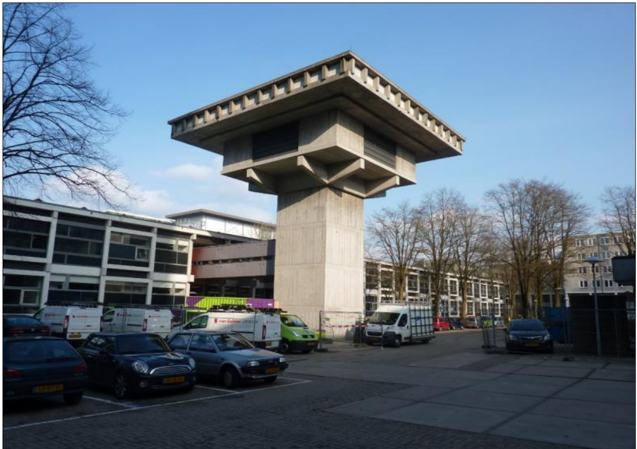
Figure 1: The Sterrentoren (photograph: David Baneke).
