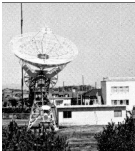
Figure 9: The 10-m parabolic antenna installed at Hiraiso in 1967 and used at 100 and 200 MHz (after Wakai, 1988).
