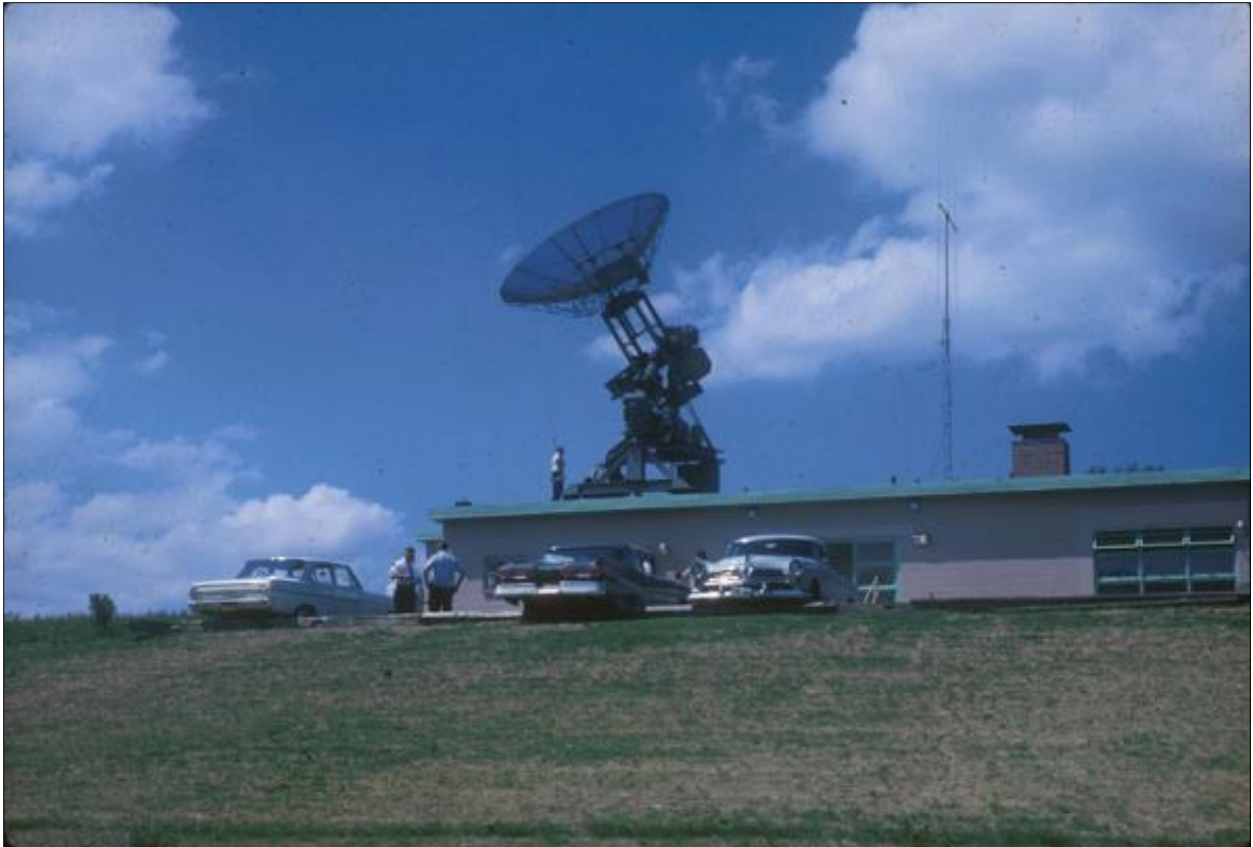
Figure 16: The new radio astronomy building at Danby south of Ithaca with the 5-m antenna on the roof (courtesy: Marshall Cohen).
