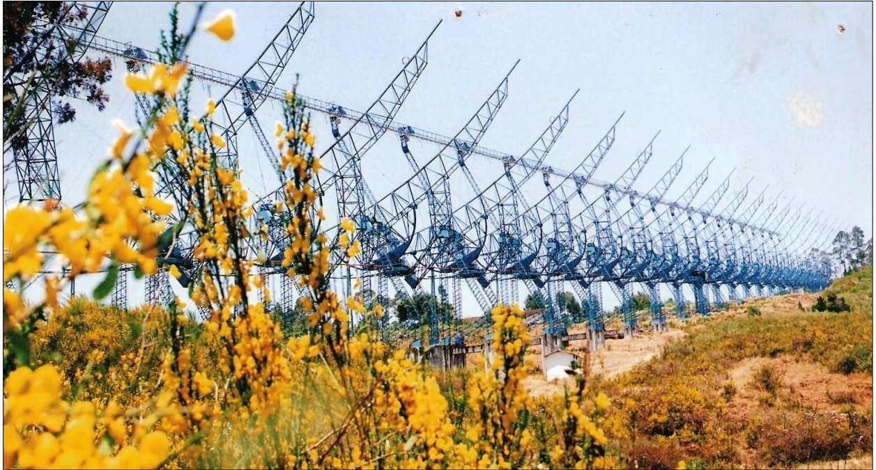
Figure 46: The Ooty Radio Telescope, consisting of the 530 m long and 30 m wide cylindrical parabolic antenna placed along a north-south sloping hillside at an angle of 11.3^\circ so that its axis of rotation is parallel to that of the Earth (courtesy: TIFR Archives).
