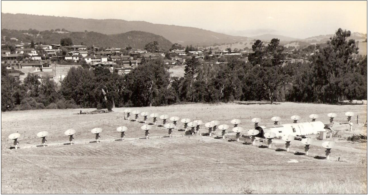
Figure 36: The completed Stanford 9.2 cm cross-antenna interferometer (courtesy: TIFR Archives).
