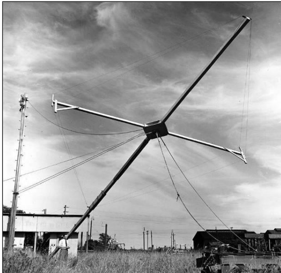
Figure 22: The rhombic aerial of the world's first radio spectrograph, at RP's Penrith field station (RAIA).
