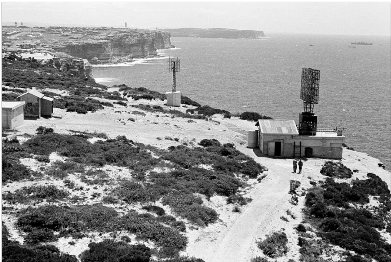
Figure 27: An aerial view of Dover Heights at the end of WWII, showing the 200 MHz radar antenna (right) used for the earliest radio astronomy observations, with the entrance of Sydney Harbour in the background (RAIA B81-1).
