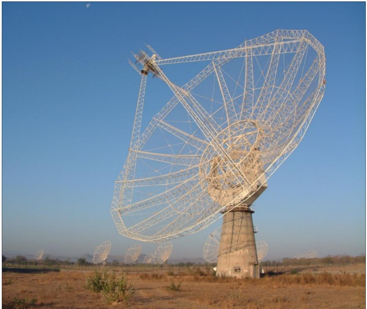
Figure 52: A close up of one of the 45-m antennas, with six others in the background (courtesy: TIFR Archives).
