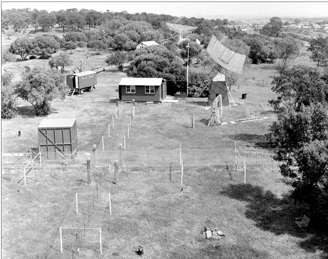
Figure 25: In the foreground is part of the prototype Mills Cross, and in the background are the ex-Georges Heights radar antenna, the 11-m hydrogen-line dish and various instrument huts (RAIA 3171-4).
